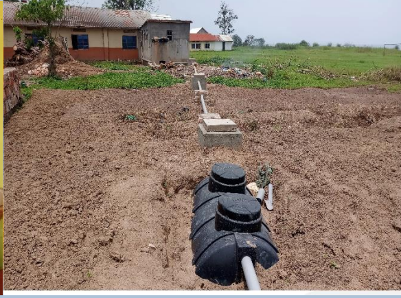
Renovation of Old Girls' toilets
