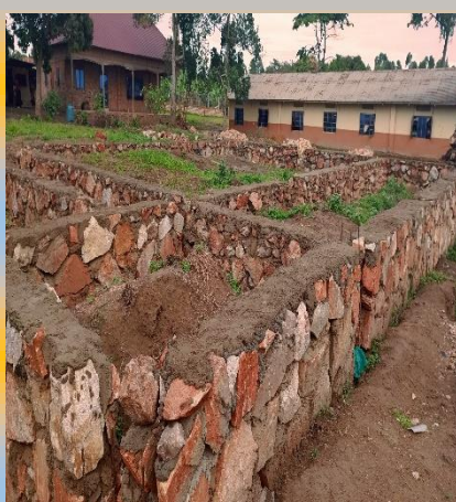
New Girls' dormitory under Construction.
